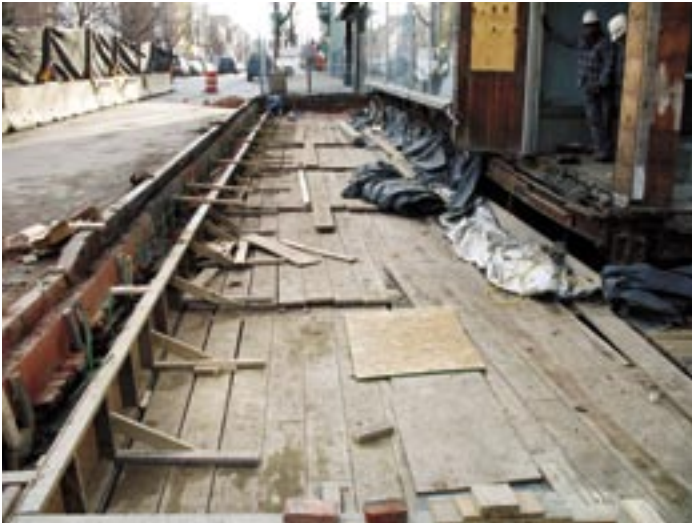
Sidewalk work at the Conservatory, downtown Troy
