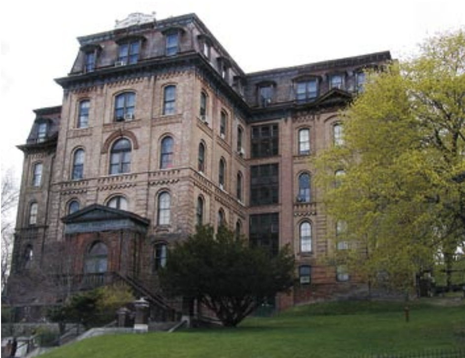
Left: South and west facades before restoration work began
