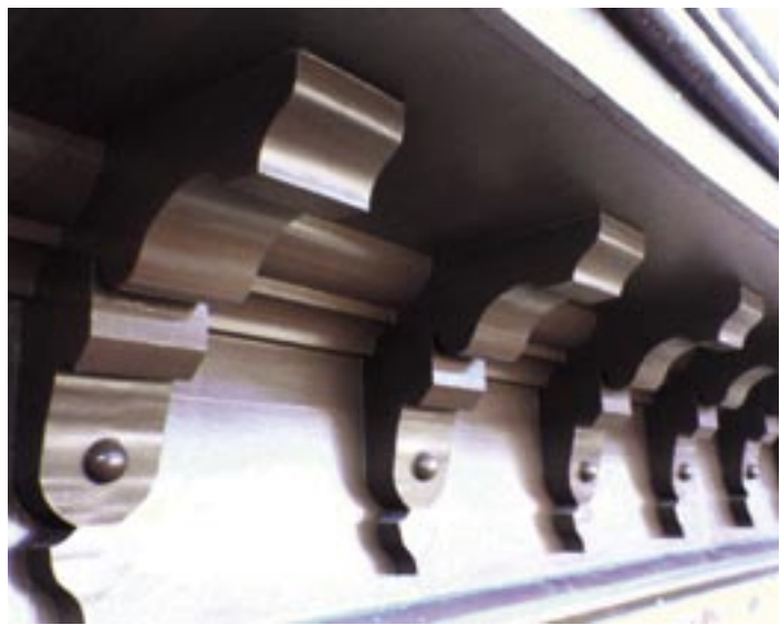
Restored cornice small brackets
