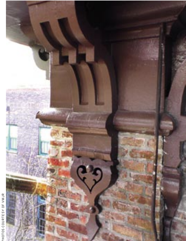
Northeast large bracket, which displays the bracket and restored masonry prior to painting.
